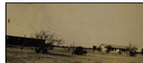
VPS Vail School Boxcar Shop Building
