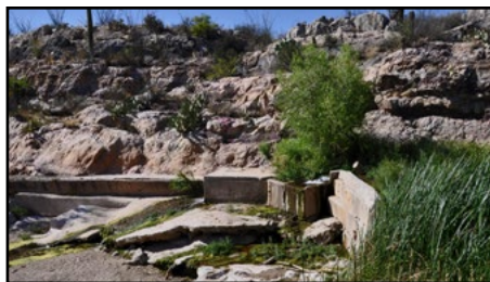
Cienega Dam looking north
