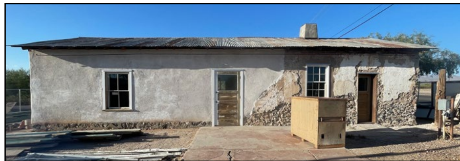
Old Vail Post Office rehabilitation. Courtesy Vail Preservation Society
